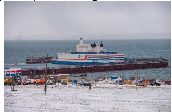
Akademik Lomonosov Floating Nuclear Power Plant
