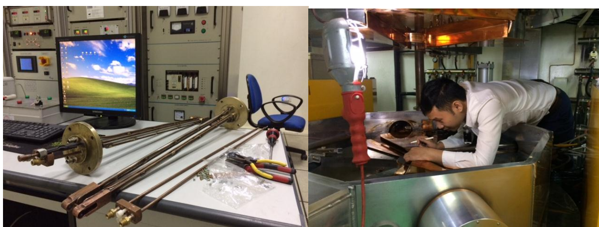
Manufacture and installation of an ion source for the KOTRON-13 Accelerator under a ministerial project
