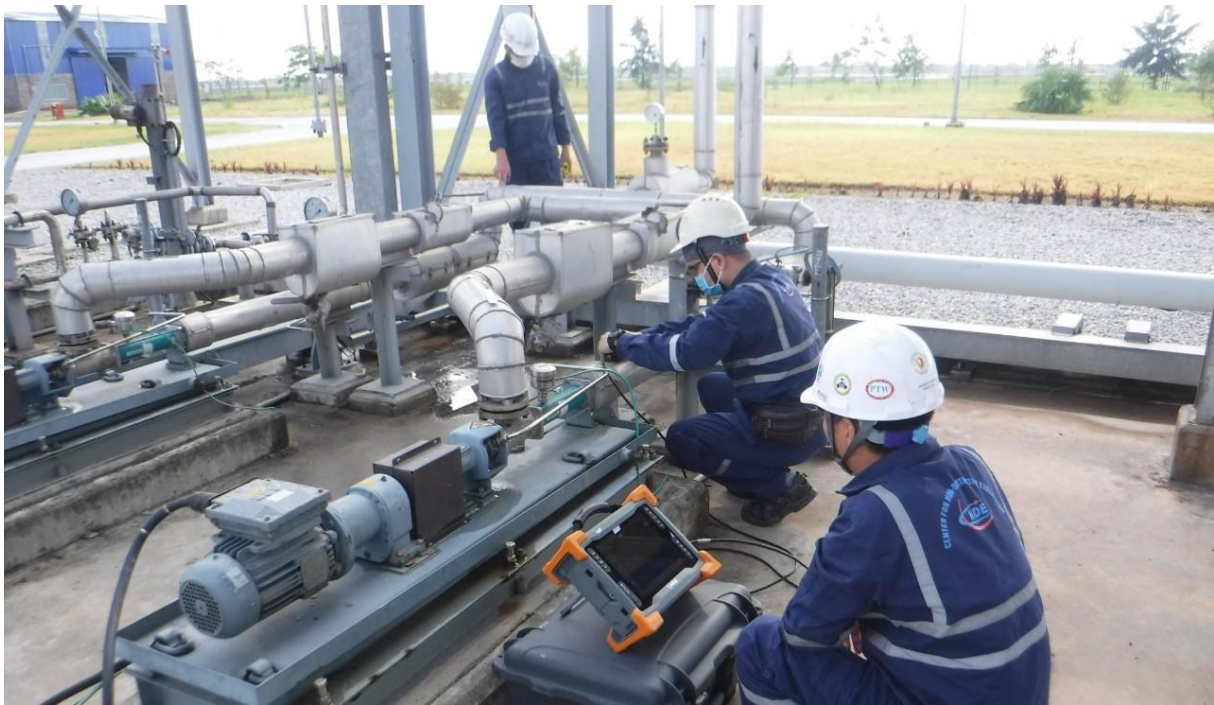
Applying the results of the ministerial-level project 2019-2020 to carry out the inspection at Tien Hai gas distribution station of Hai Phong gas branch, Vietnam gas corporation
